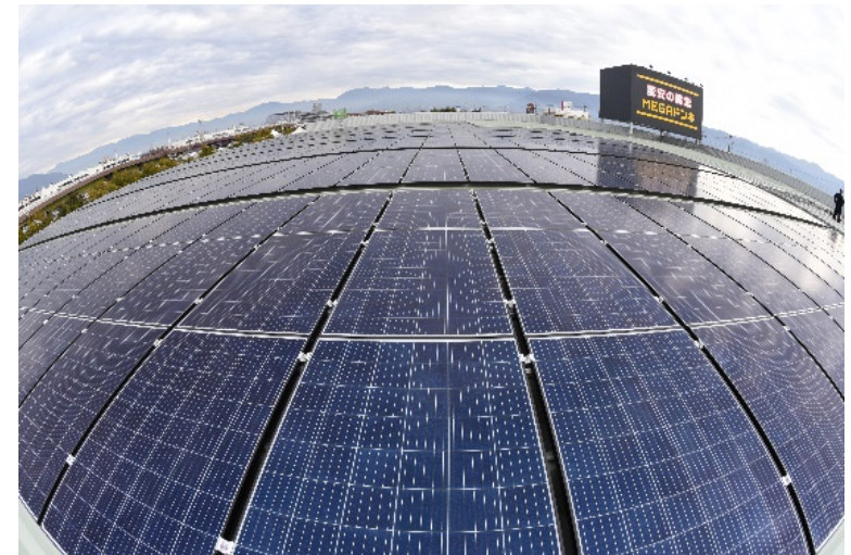
solar panels (MEGA Don Quijote Kofu)
