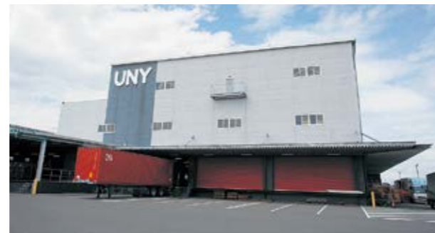
Recycling center at Yatomi Distribution Center
